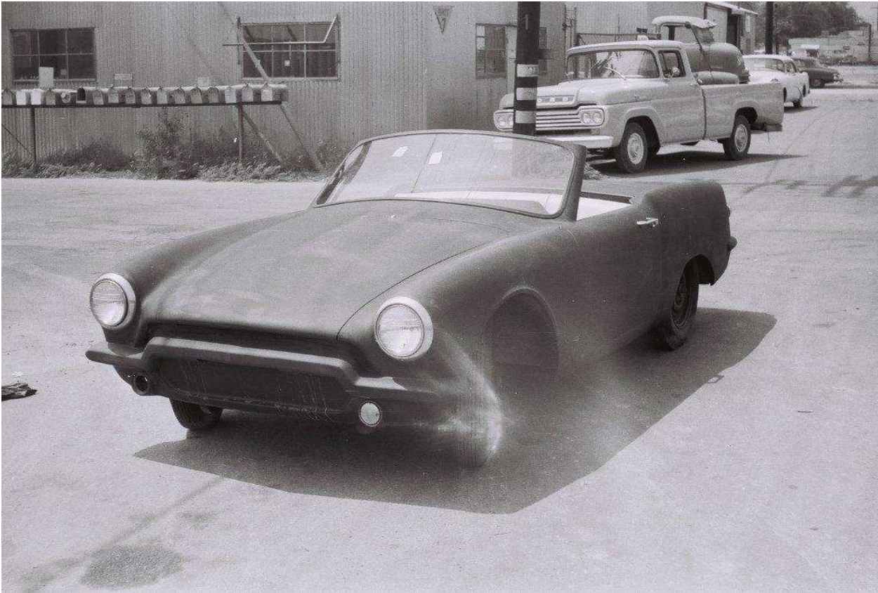
The final Pioneer Electric Design - maybe it still exists, notice the VW axle
